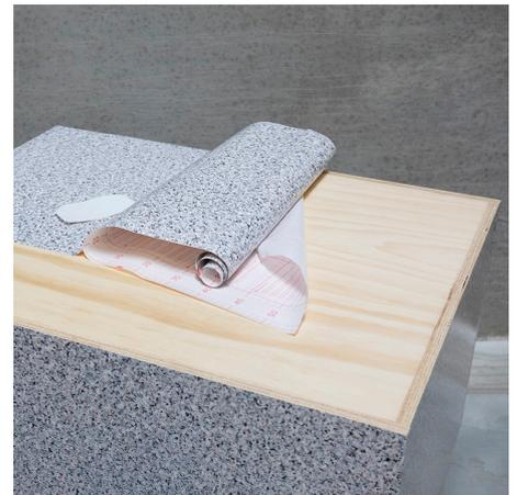
**9** The self-adhesive film fits across the width of the 45 cm wide podium. Start with the sides and make sure to start away from the edge on one side, so that the foil can overlap. Finish with the top board; attach the foil 2 cm over the sides so that you can cut a notch for the corners to be stuck down over the sides.
