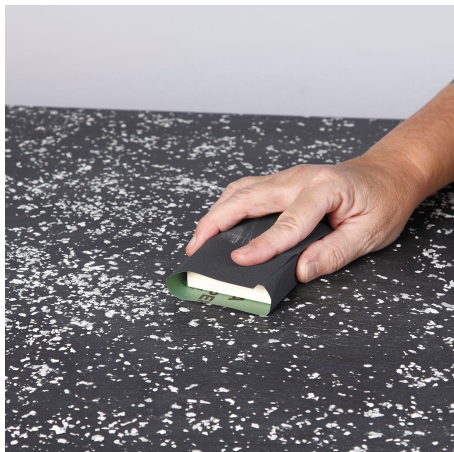
12 Sand the surface lightly with sand paper.
